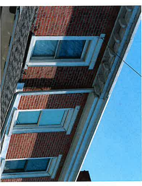
Note the original brackets on left and the inappropriately covered brackets on right.
