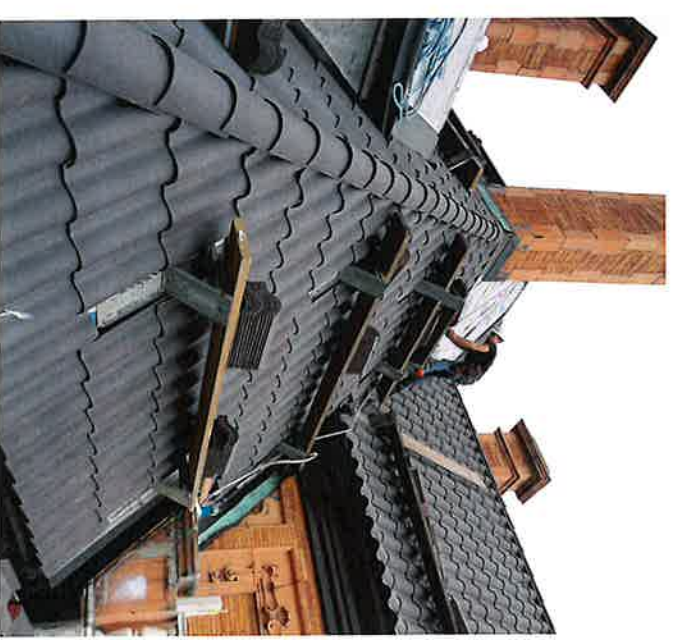
This replacement historic terra cotta tile roof should last 100 years.
