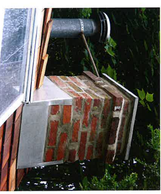
Poor Flashing: Covers too much of historic chimney.
